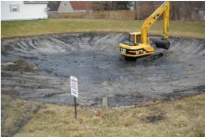
Figure 2: One of the Foxwood Villa stormwater ponds in the midst of a dredge operation (City of Toledo Engineering Service 2015)
